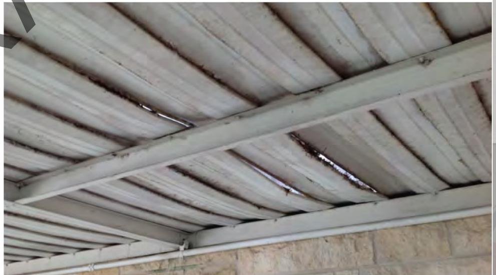
Figure 8-1. The Canopy around the Golf Course Club House. You can see the deterioration and damage that has happened due to weathering.
