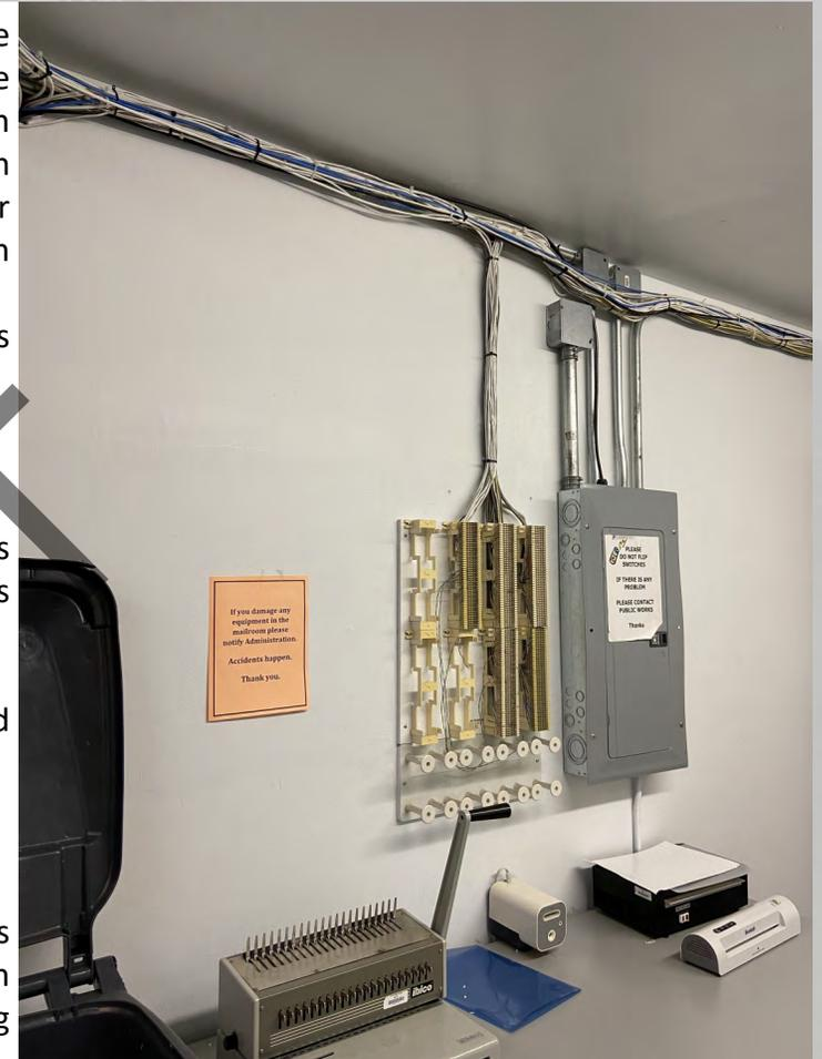
Figure 8-3. Exposed wiring in City Hall
